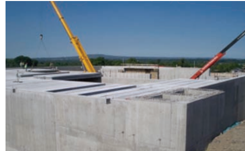
Longford Central Regional Water Supply Scheme stage 6
